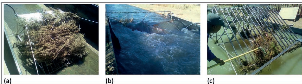
Figure 20. Debris blockage (a) during maintenance period (b) major debris build up after a 2-week interval (c) turbine removal and cleaning at 2-week interval
