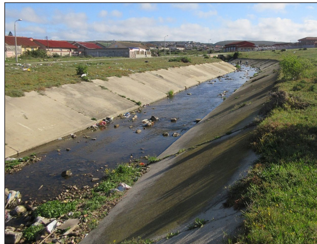
Figure 4. Trapezoidal channel used for the collection of flow data
